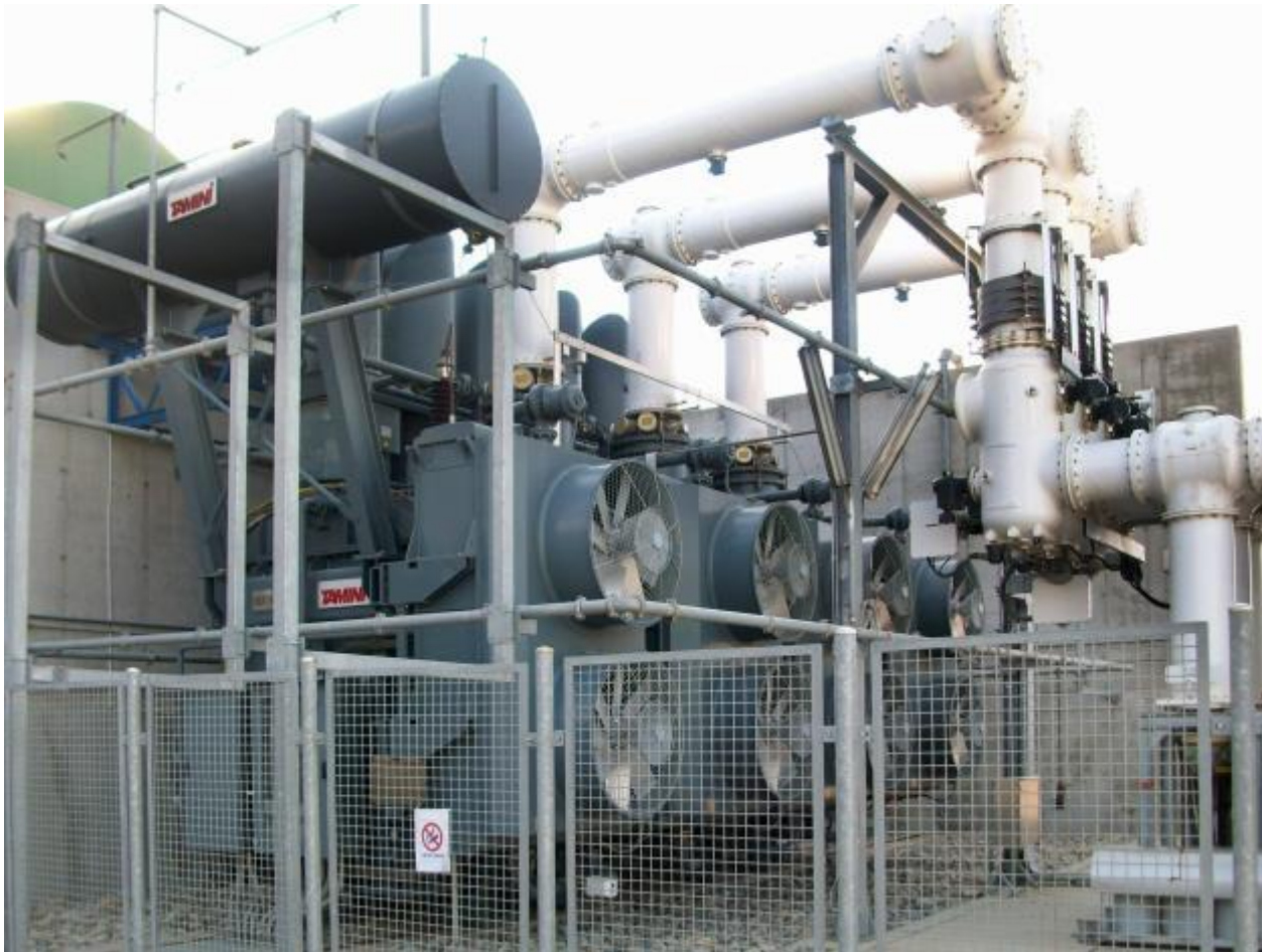
TECHINT/SCANDALE – Power Transformer 553 MVA, 403/19/15,75 kV
