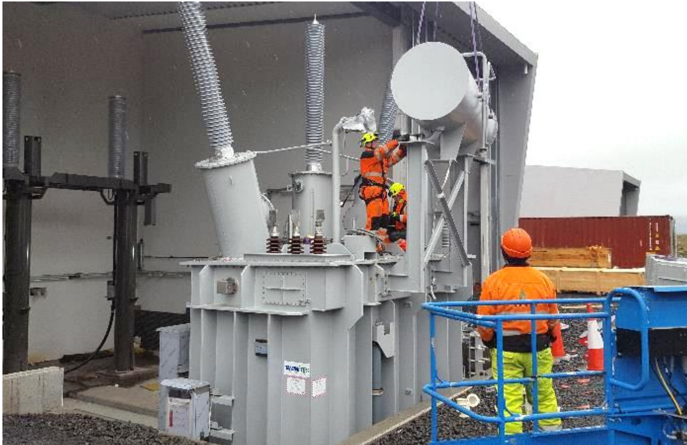
LANDSVIRKJUN – N.4 Power Transformer 50 MVA, 220 kV for a Geothermal Power Station in North Iceland
