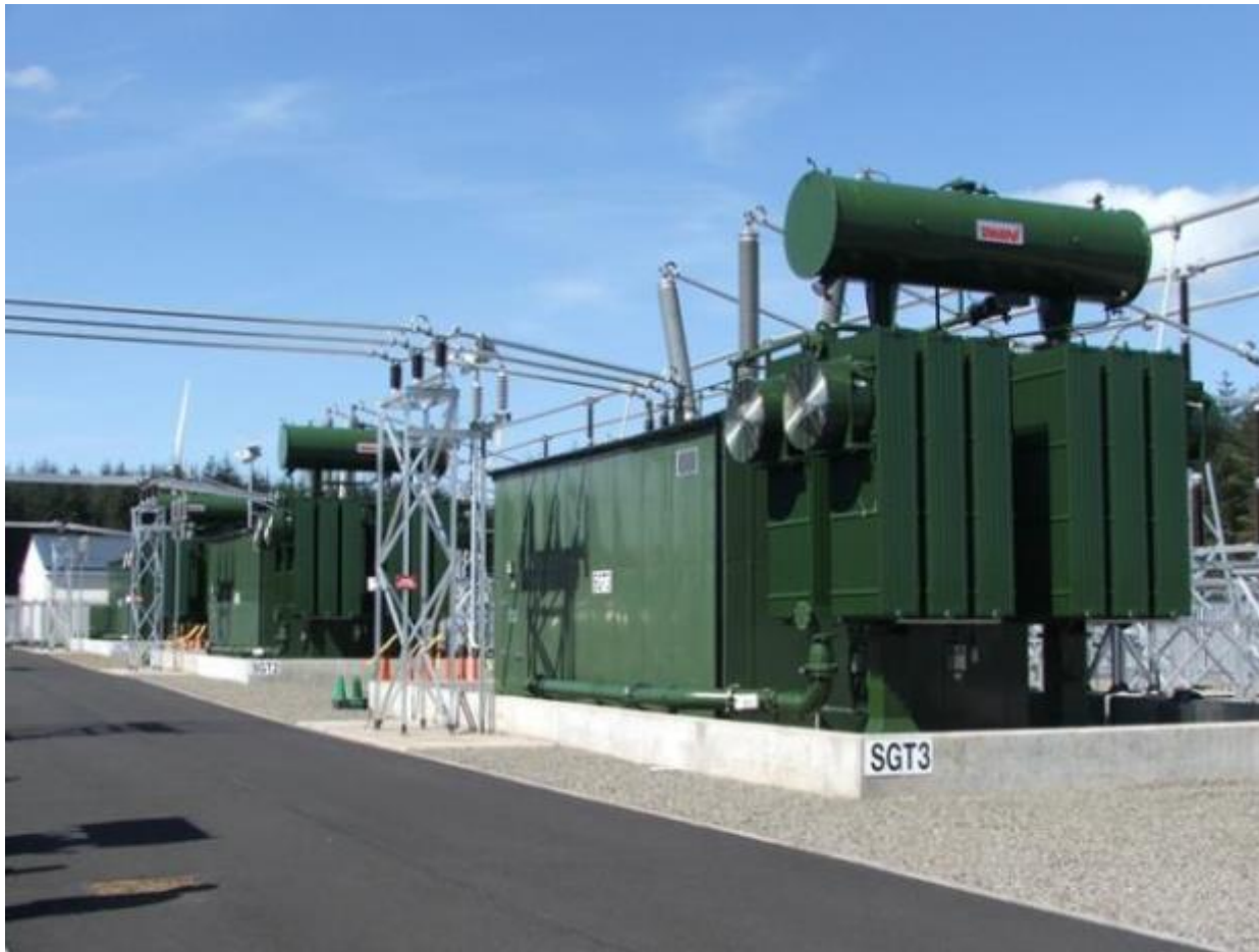
Substation Transformer 120 MVA, 275/33 kV Scottish Power - Whitelee Windfarm (GB)
