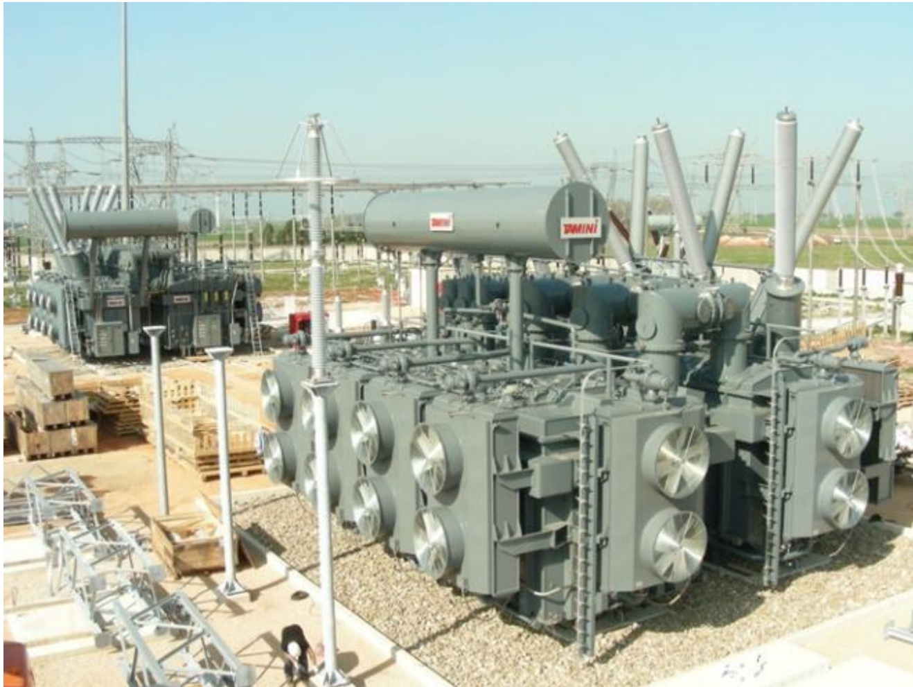
TERNA - PST 1.800 MVA, 400 kV ( \pm 17.5 )
